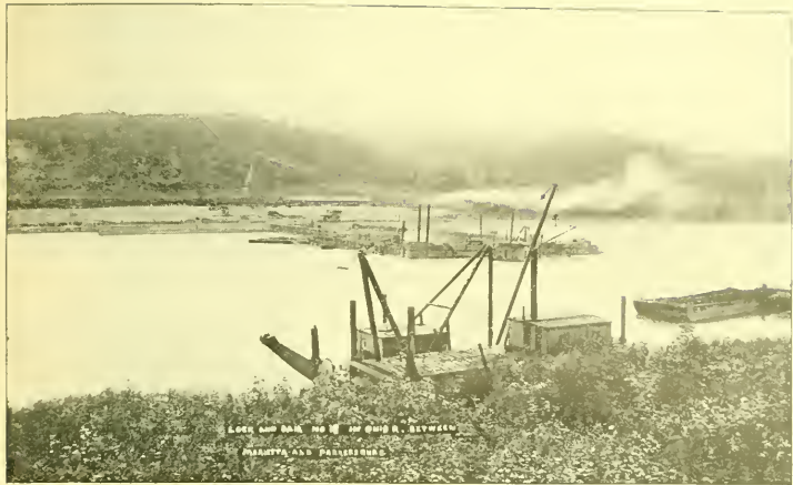
Lock and Dam, No. 18, Parkersburg, W. Va.
